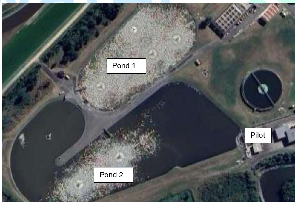
Figure 2: Totara Rd. Wastewater Treatment Plant in Palmerston North
